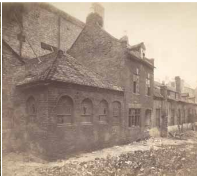
Baskerville's type foundry in Birmingham on the eve of demolition, 1887.
