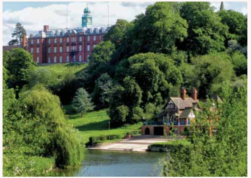
Shrewsbury School, formerly a branch of the Thomas Coram Foundling Hospital.
