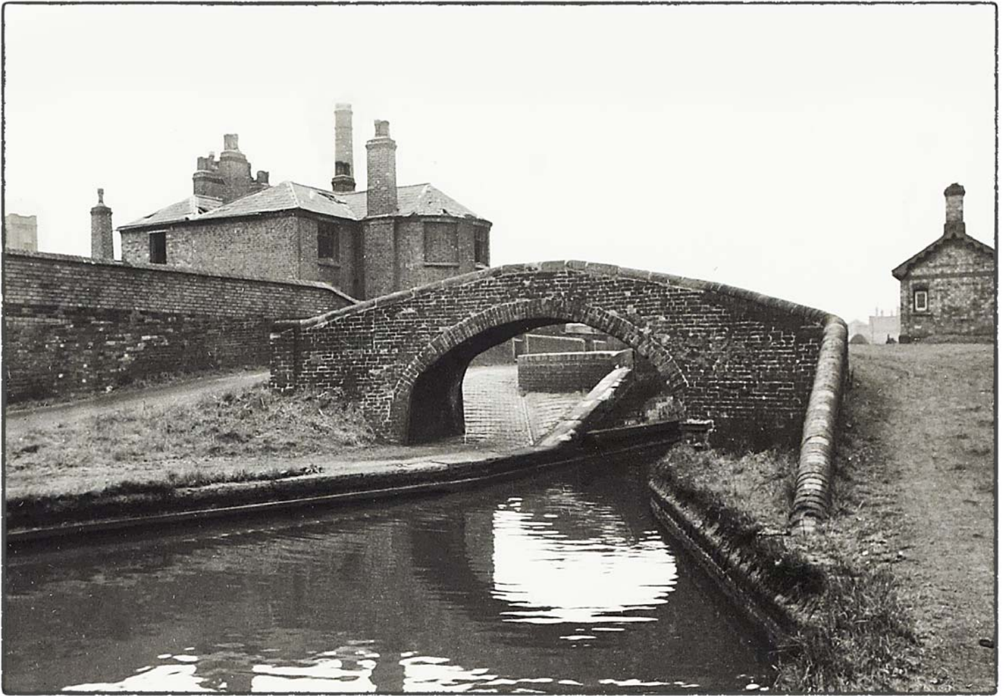
The Smethwick top lock, lock house and toll house.
