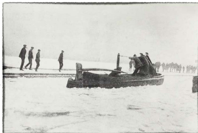
Men working on an ice boat near Conduit Colliery on the Birmingham Canal Navigations c.1920.
