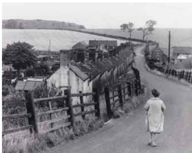
A settlement of miners cottages in Dark Lane, Malinslee, 1962. These were demolished to make way for Telford new town.
