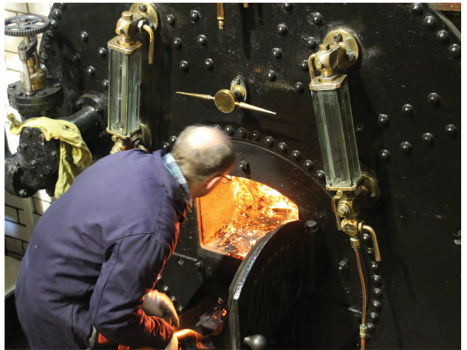
Firing up the boilers at Coleham Pumping Station, Shrewsbury. The coal-fired boilers drove the two beam engines which formed part of Shrewsbury's sewerage system.
