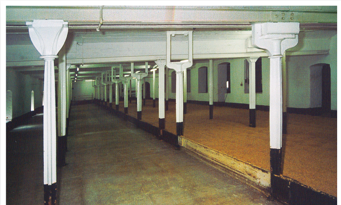
Ditherington Mill. Three lines of cast-iron columns run along each floor, supporting cast-iron beams. Each beam is cast in two halves which are bolted together through heavy flanges.
