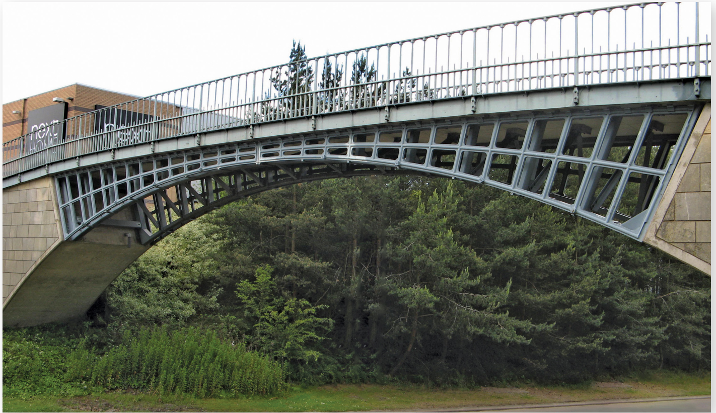
Hazledine's arch ribs reused in Telford Town Centre.
