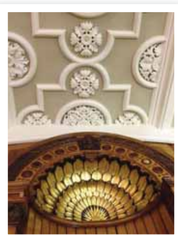
Detail of the newly restored Shakespeare Memorial Room
